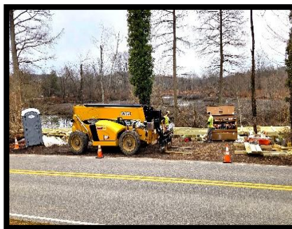
Winter 2026 Construction Parking Lot
